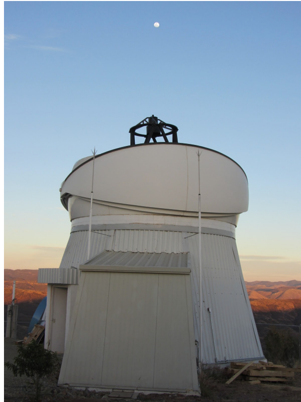
Figure 1. The TIGRE facility at La Luz Observatory.
